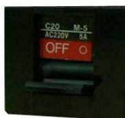
Power switch (breaker)
